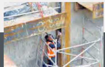
Onsite welding in New Lynn Railway trench.
